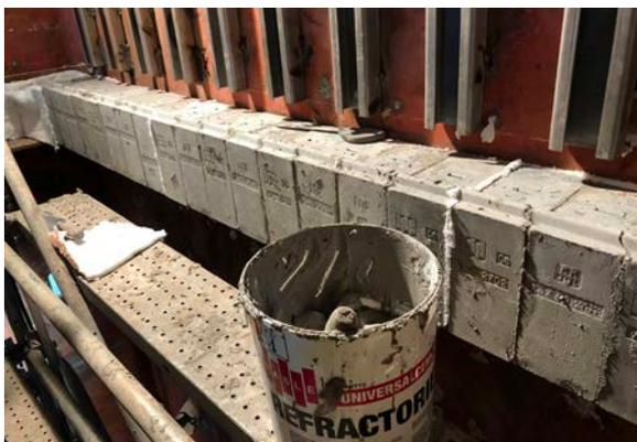
**Steel rails are welded onto the casing and HASLE's console lining is installed with mortar between the elements. It is now ready for installation of the precast Modular Lining elements.**
