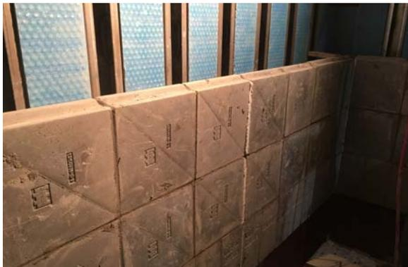
**Precast elements are installed on the steel rails, on top of the console elements, with vermiculite back-up insulation between the rails. Ceramic fibres are installed between every four elements (every 1 m) to allow thermal expansion. Now, the system is only missing the pouring of the insulating castable behind the pre-cast lining.**
